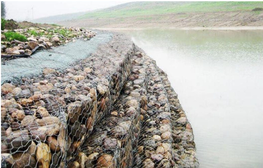
Figure 2.1: Gabion Retaining Wall
